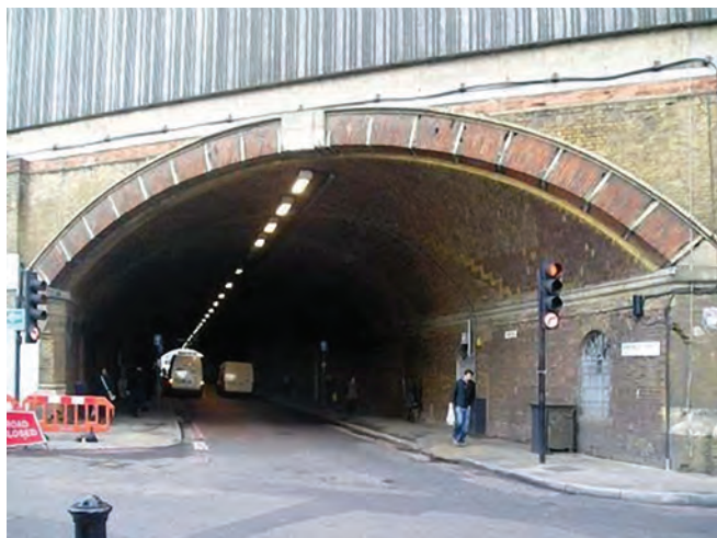
View of the Bermondsey Street tunnel under London Bridge railway viaduct, taken in 2012 before all the reconstruction work in the vicinity
